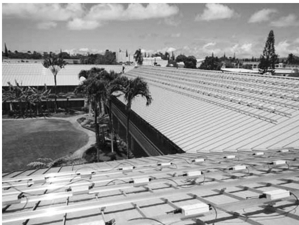
Figure 6: Installation where all roof orientations are used
